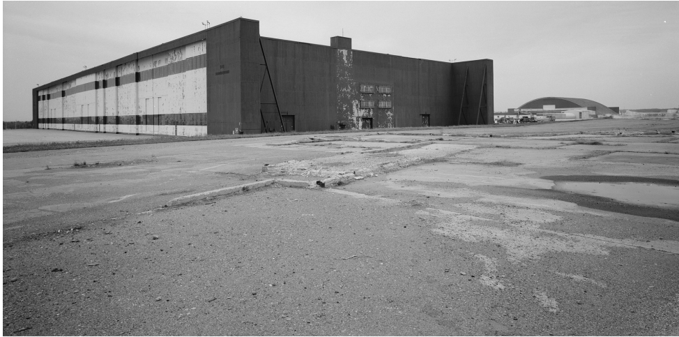
Loring Air Force Base Double Cantilever Hangar. Historic American Engineering Record.
